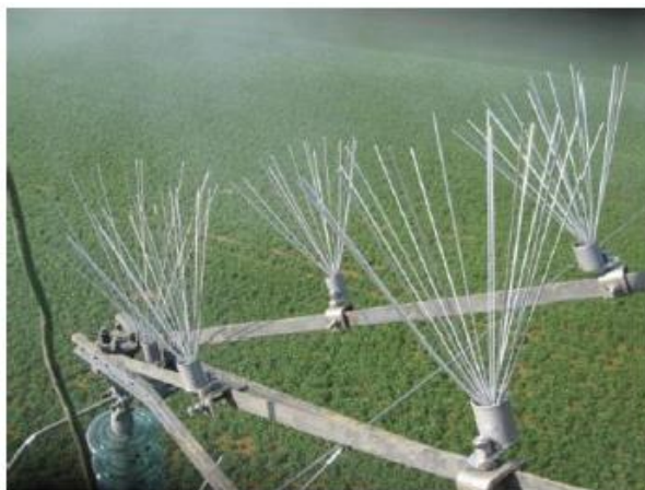
Figure 7-7: Anti-nest device (RTE, 2014)
