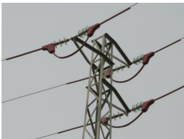
Figure 7-7: Anti-nest device (RTE, 2014)
