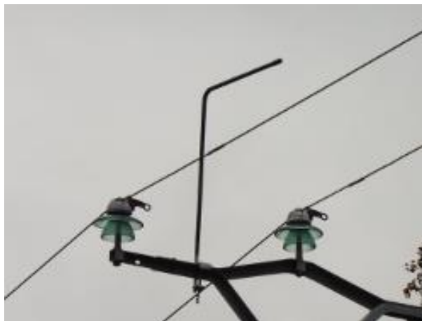
Figure 7-8: Perch installed on a pylon (Enedis, 2016)
